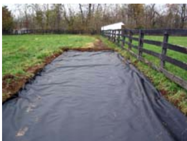
Figure 3. Geotextile fabric in place after excavation.
