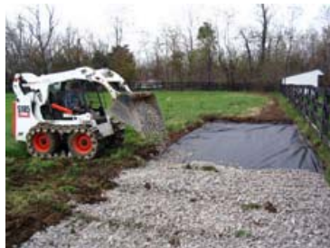
Figure 5. Base layer of crushed stone.
