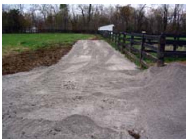
Figure 7. Surface layer of crushed stone
